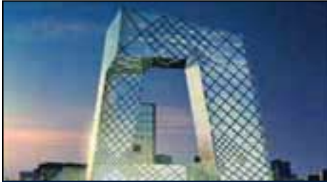
China Central Television's new Television Cultural Center, designed by Rem Koolhaas.
